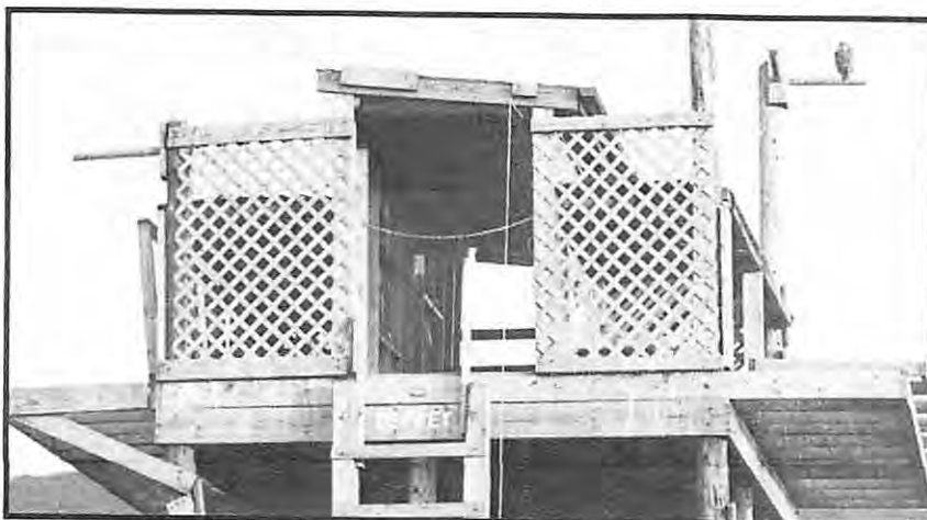
The hacking tower platform
