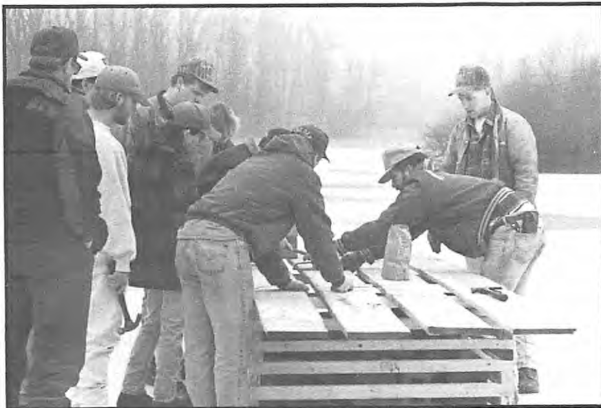
PA College of Technology students build fish cribs on ice-covered Fish Commission ponds.
