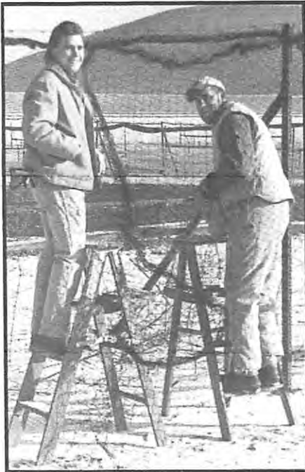
Arron Lyons (l) and Mark Knapp repair flood-damaged pheasant-rearing pens.
