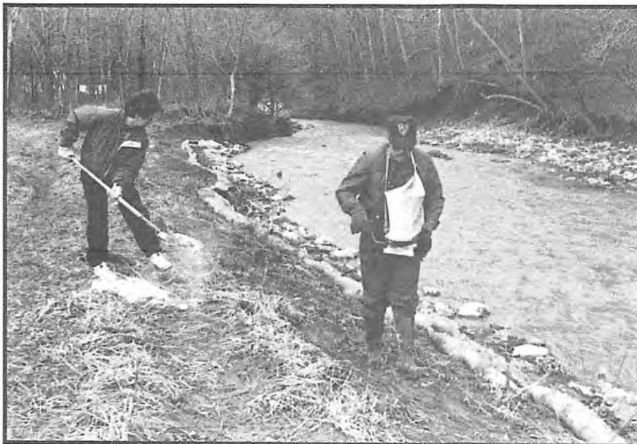
Maryland DNR and NRCS employees work side by side liming and seeding a portion of streambank in the Town Creek Watershed.
